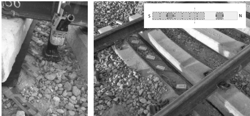
FIGURE 8 Installation and location of the sensors at the ballast-tie interface
