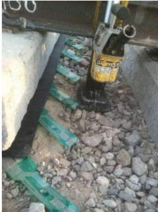
Figure 7.5 Pressure sensors being installed under raised track
